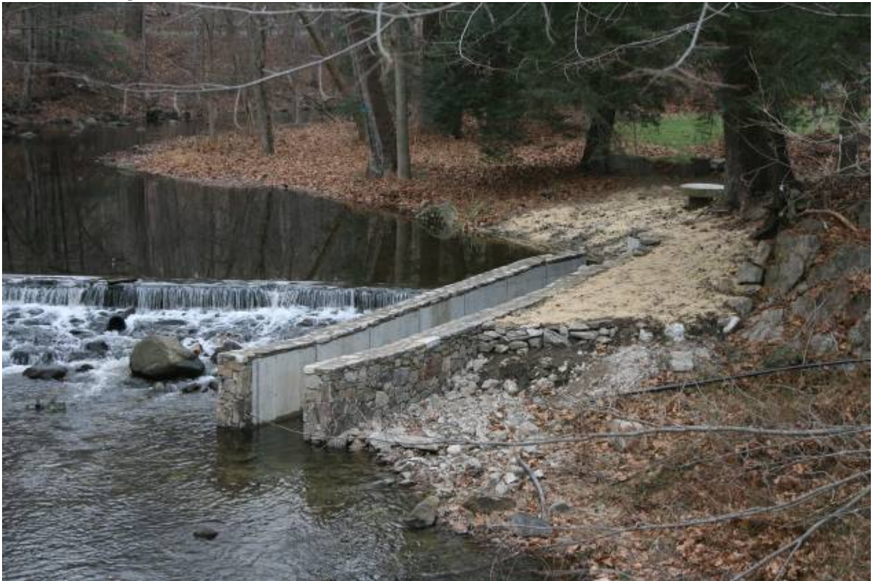
Low Dam before (top) and after fishway construction (above). Photos courtesy of Sally Harold.
