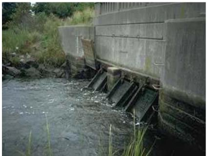
FIGURE 1-3. One of Four Flap Tide Gates Open at Hammock River
