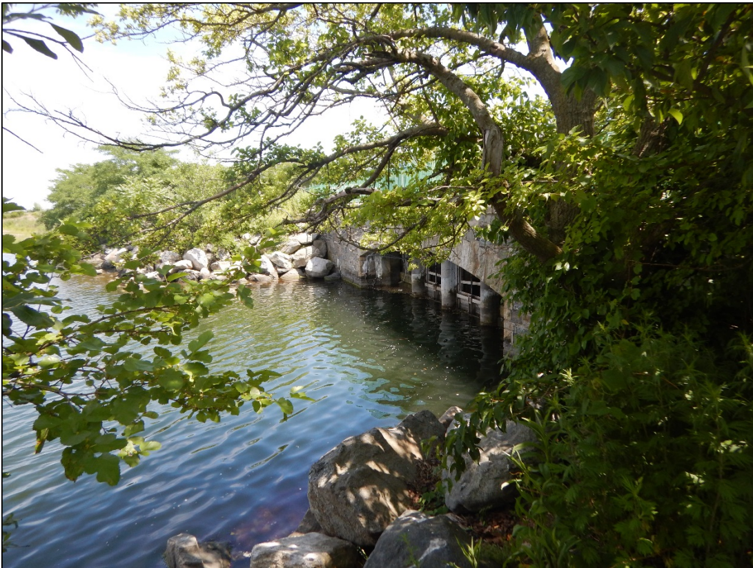
View of the tidal gates at Manursing Lake ( photo NYSDEC ).
