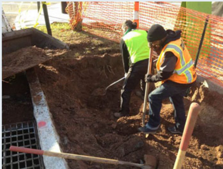
Urban Resource Initiative's GreenSkills crew building the first of eight residential bioswales to divert stormwater runoff in December 2014.
