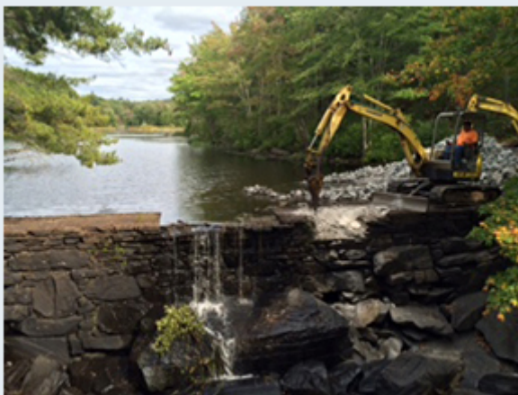
The Ed Bills Dam in Lyme, CT, as it was being removed.
