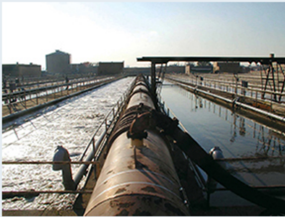
Hunts Point Sewage Treatment Plant: 42" sludge pipe at West Aeration Tanks (looking west). Photo by NYC Dept. of Environmental Protection.
